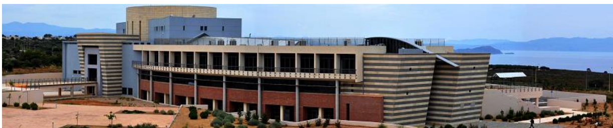
Figure 1 ECE Department Building, Kounoupidiana Campus, Technical University of Crete (TUC), at Chania, Crete, Greece
